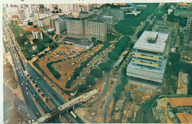
5.6.2 — Significant Expansions and Restoration
